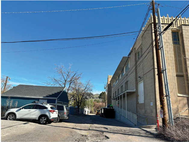
ALLEY VIEW LOOKING NORTH
